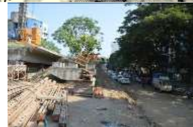
Flyover under construction
