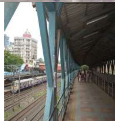
Existing F.O.B and Railway Station.
