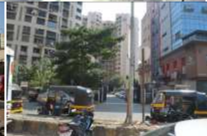
Existing building structure, Maple and Morya Buildings.
