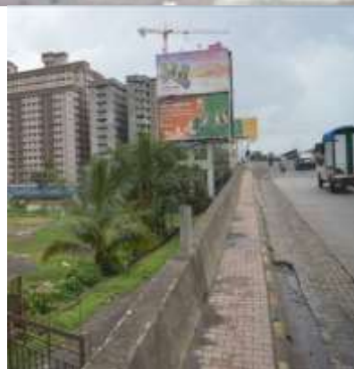
Existing flyover with existing building.
