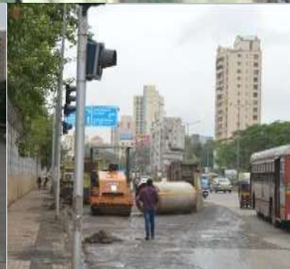
Existing service road.
