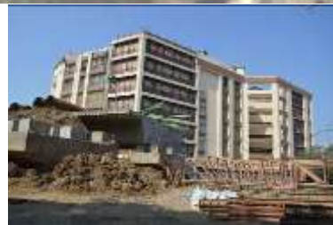
School building adjacent to site
