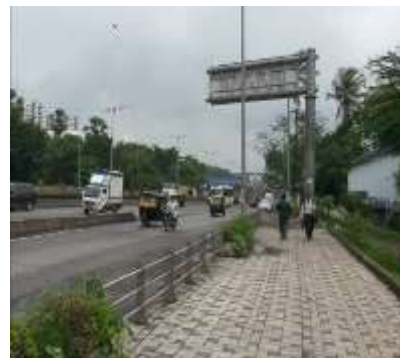
Existing road with footpath.
